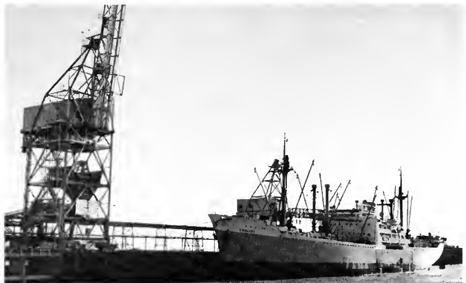
Dry bulk materials handling plant at Port of Houston.
